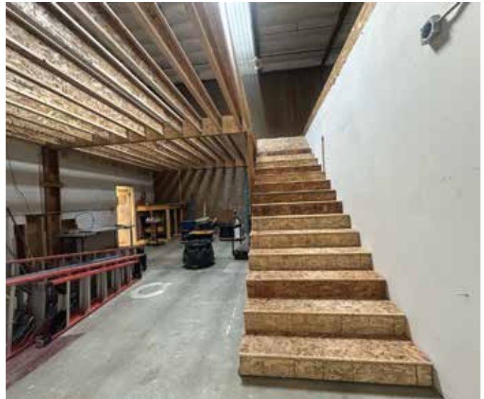
Verge studio construction, 2025.
